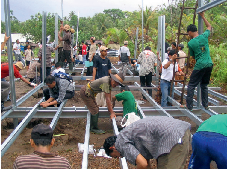
Community involvement is the foundation for community based psychosocial interventions
